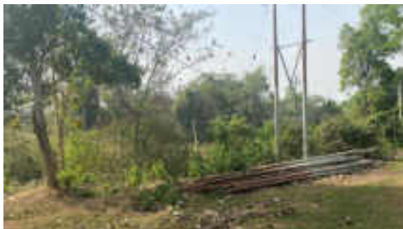
Storage of poles along roadside in Gamitila – Kalyanpur distribution line route
