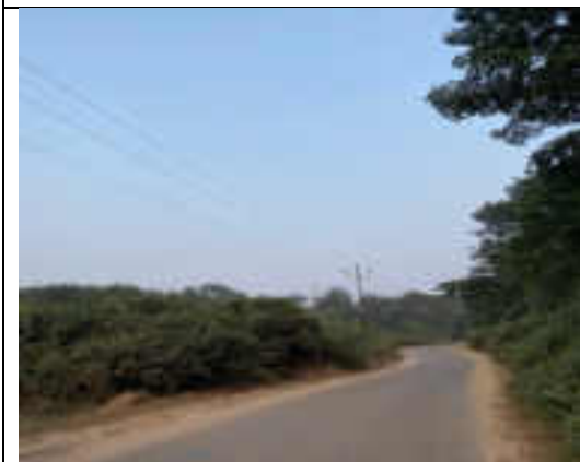
Gokulnagar Substation to 33 kV Madhupur Substation
