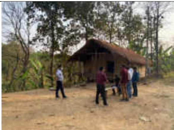
4. Tribal hut below Distribution Line (132 kV Mission Tilla Substation to 33 kV Dhamchara via Panisagar Substation) with risk wire falling on roof and electrocution/fire
