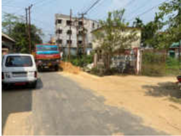
6. 33 kV UG from Grid Sub Station to College Tilla Substation route showing potential health risk during construction, when road will become congested and students' movement (school gate shown)
