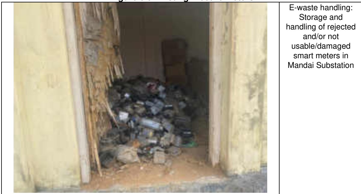
Figure 5.9 Existing Electric Meters
