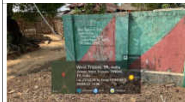
Water storage built by Mandwi Forest Range in ESD Mandwi
