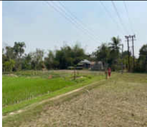
9. 33 kV UG from Grid Sub Station to College Tilla Substation route- potential pole topple/wire snapping on fields during monsoon.
