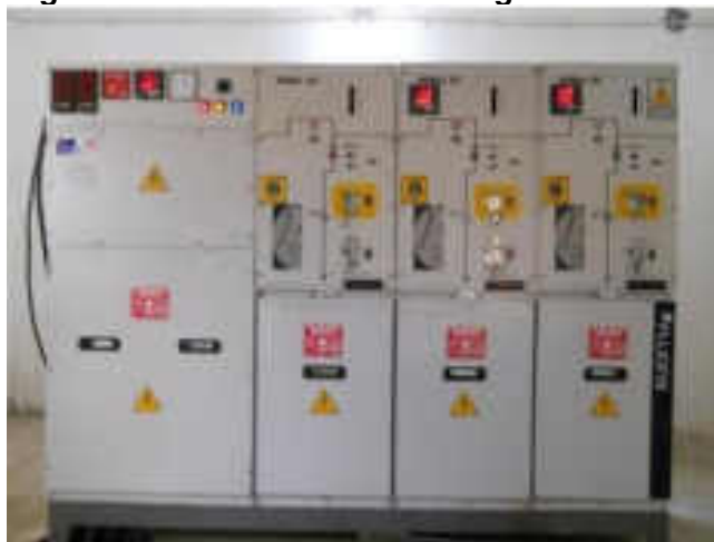
Figure 3.4 Illustrative 12 kV Ring Main Unit
