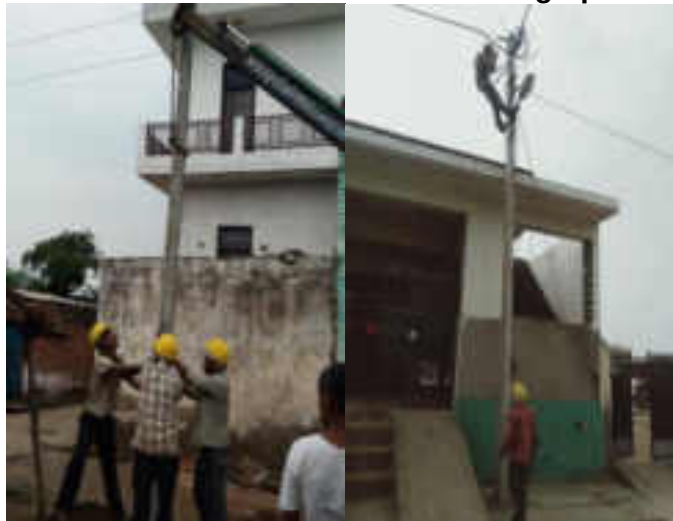
Figure 3.19 Representative Under Construction Photographs of ABC Installation
