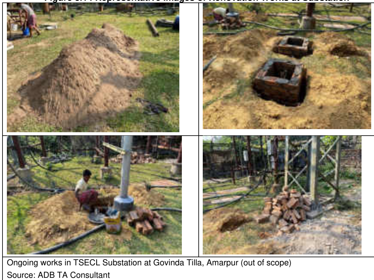
Figure 3.14 Representative Images of Renovation Works at Substation
