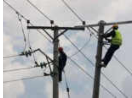
Figure 3.18 Representative Under Construction Photographs of Covered Conductor Installation
