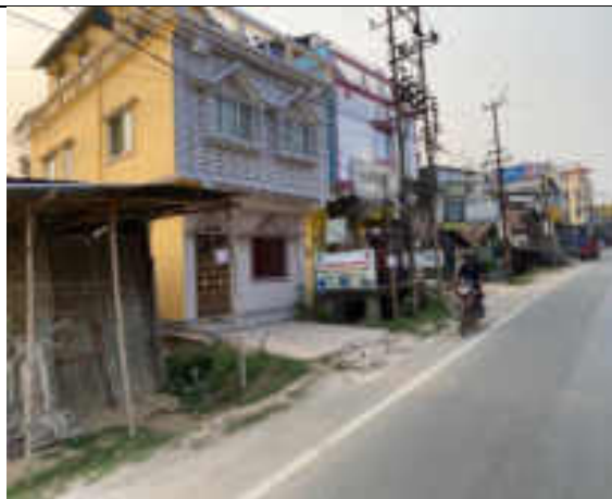
11. 11 kV (UG) Milan Chakra Feeder from Badhaghat Substation to CNG Station route showing- UG ROW route
