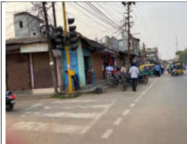
10. 11 kV (UG) Milan Chakra Feeder from Badhaghat Substation to CNG Station, showing- UG ROW route
